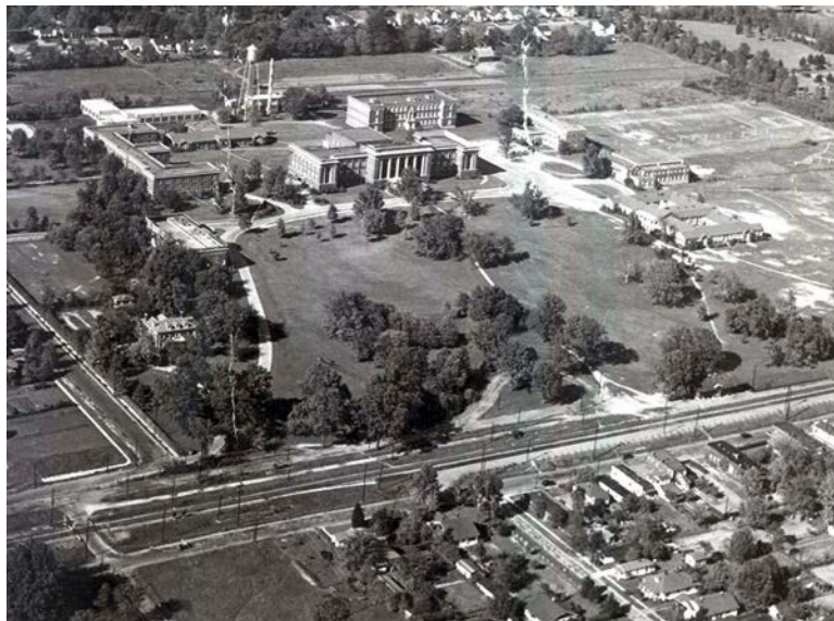
Figure 2.3. Normal Station rail stop in early 1900s
