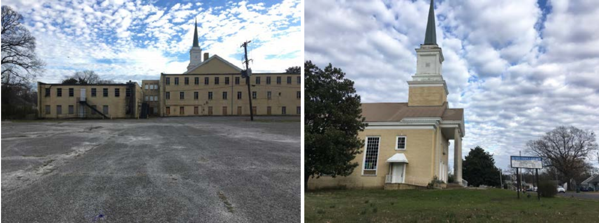
Images 2.13 and 2.14. Bethel Temple Church boarded windows in annex buildings (left) and street front chapel (right)
