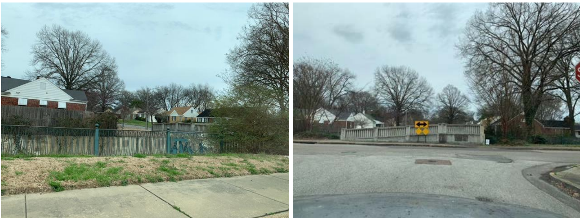
Images 2.23 and 2.24. Pedestrian infrastructure providing access across Black Bayou (left and right)
